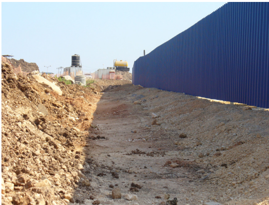
Figure 12: Storm water run-off prevention during construction
