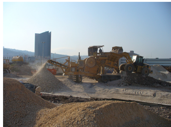
Figure 14: Rock waste crushed on site and recycled
